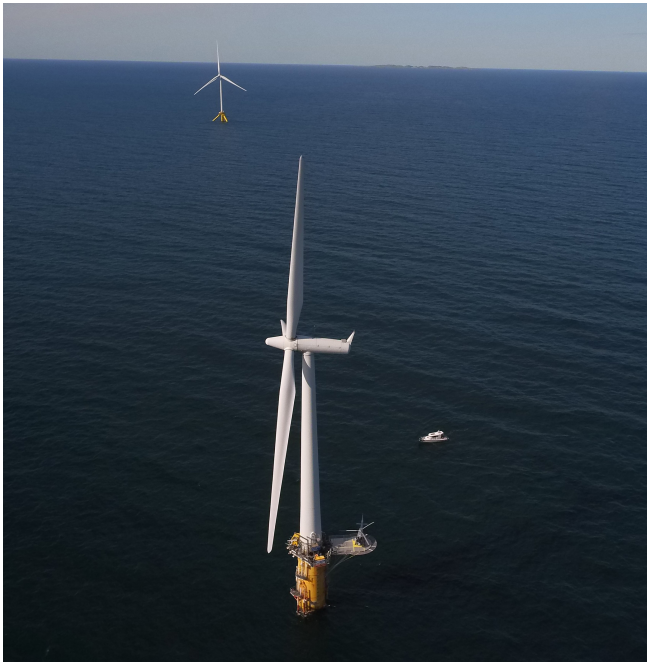
Figure 5. The Zefyros floating offshore wind turbine relies on a Siemens 2.3 MW device. Credits: Unitech Energy Group
