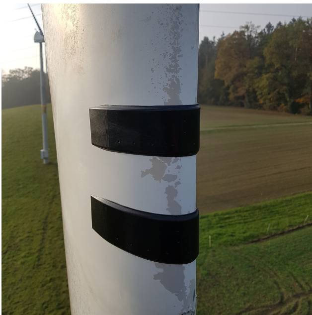
Figure 5. PolyJet 3D-printed housings glued on a 6 kW operating wind turbine to test its robustness.
