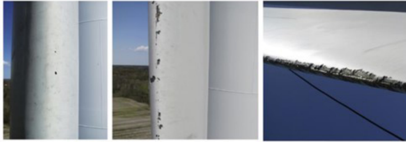
Figure 19. Changes to the LE surface due to impact with a different degree of severity. From left to right, LEE at an early stage, severely damaged coating and LEE starts to wear the shell material. Adapted from Keegan et al. (2013) and Rempel (2012).
