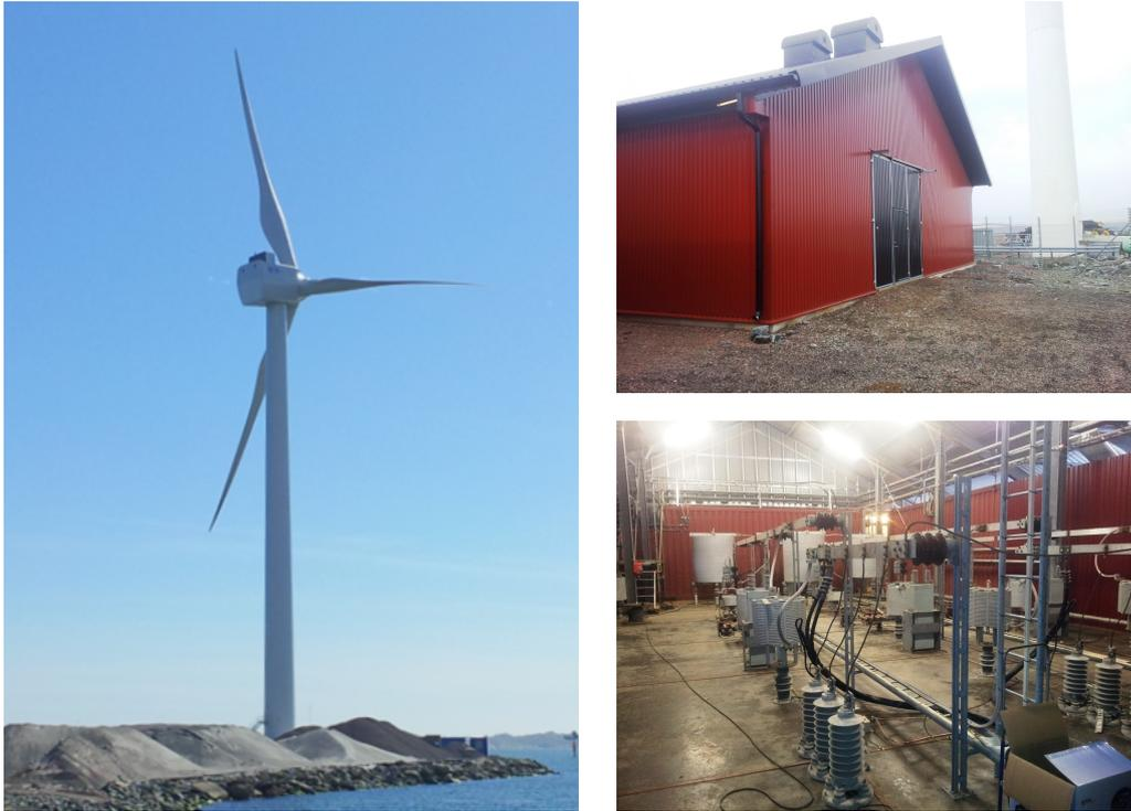
**Figure 3.** Testing facility in Gothenburg test facility, comprising the 4.1 MW FPC “ÖCfBig Glenn” ÖCØ wind turbine; housing of. The facility houses the back-to-back HVDC station, and coupling inductor (back) and AC filters (front) inside the house.
