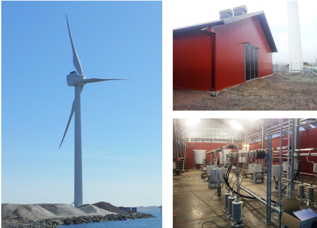
Figure 3. Gothenburg test facility, comprising the 4.1 MW FPC “Big Glenn” wind turbine. The facility houses the back-to-back HVDC station and coupling inductor (back) and AC filters (front).
