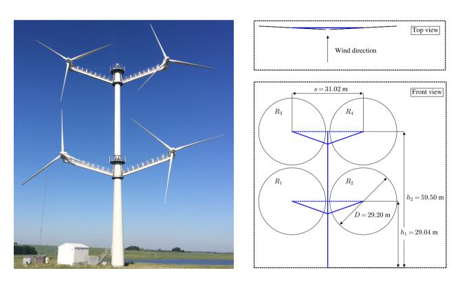
**Figure 1.** Left: 4R-V29 wind turbine located at the Risø Campus. Right: sketch of 4R-V29 wind turbine including dimensions and rotor definitions shown in a top and front view.
