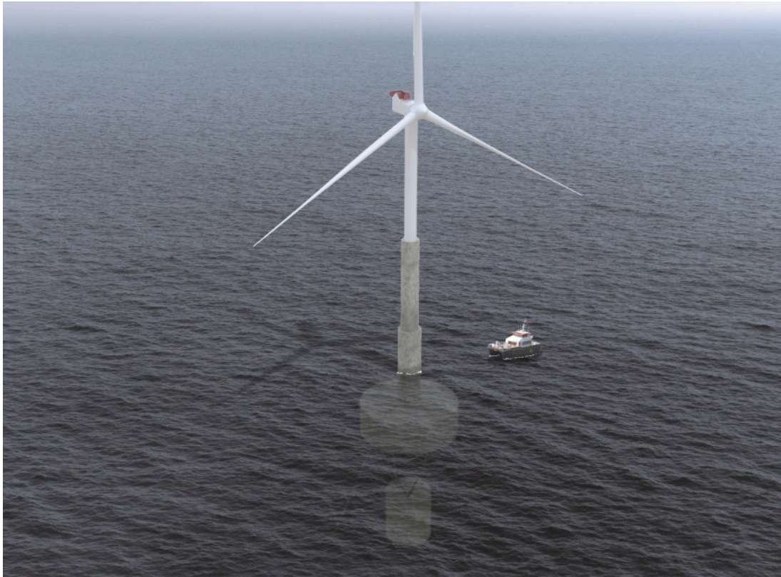
Figure 4. TELWIND® platform. Source: Figure courtesy of Esteyco [22]
