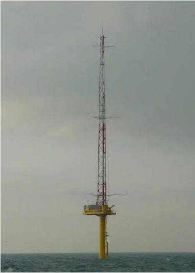
Figure 1: Meteorological Mast IJmuiden
