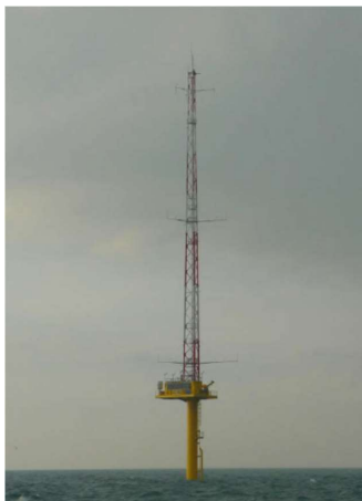
Figure 5: Meteorological Mast IJmuiden
