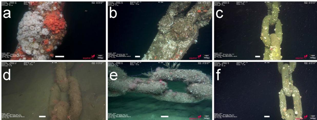
Figure 7 Example images along a typical Mooring Line (Turbine HS01's Mooring Line 111) top to bottom. a. Top Chain, Bridle Chain. b. Top Chain, Triplate. c. Top Chain. d. Middle Chain, on the seabed. e. Middle Chain, off the seabed. f. Top Chain. Scale bar = 10 cm.
