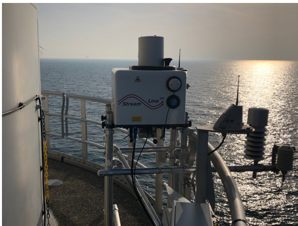
Figure 2. Long-range scanning lidar and additional measurement systems (on the right side) on the TP of one of the northernmost wind turbines (K01) at the wind farm Gode Wind 1.
