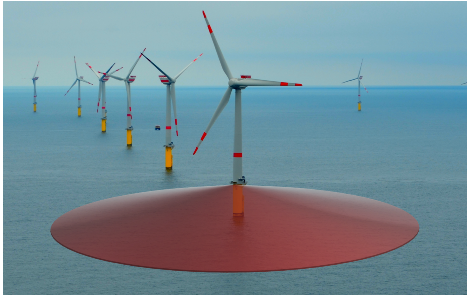
Figure 3. Schematic representation of the Sea Surface Leveling Scan Sea Surface Leveling Scan from the transition piece platform of a turbine at the Global Tech I wind farm.
