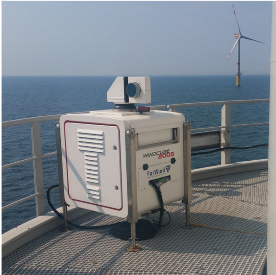
Figure 7. Image of the WindCube200S installed on the transition piece of the wind turbine in the offshore windfarm Global Tech I. Picture taken by Stephan Voß.
