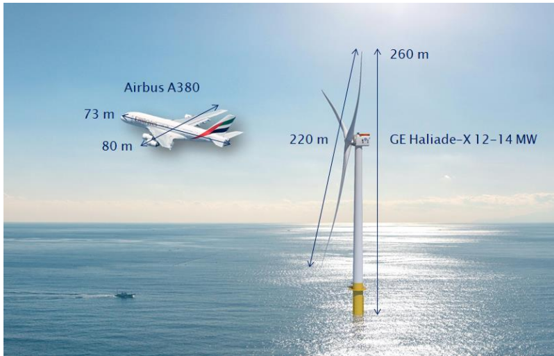
Figure 2: Modern wind turbines are the largest rotating machines on Earth. It takes three A380s, the largest civil transport airplane in the world, to span the rotor diameter of a large offshore wind turbine. Different from airplanes, however, these machines are designed to operate in a fully autonomous manner in harsh environments, with minimum maintenance while ensuring high availability, accumulating about 100 million fatigue cycles throughout their 20+ year lifetimes. (Haliade-X rendering from www.ge.com ; A380 rendering from www.airbus.com )
