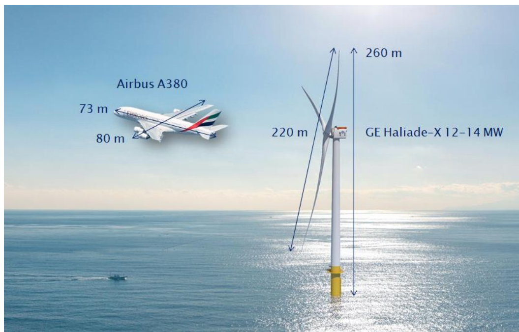
60 Figure 2: Modern wind turbines are the largest rotating machines on Earth. It takes three A380s, the largest civil transport airplane in the world, to span the rotor diameter of a large offshore wind turbine. Different from airplanes, however, these machines are designed to operate in a fully autonomous manner in harsh environments, with minimum maintenance while ensuring high availability, accumulating about 100 million fatigue cycles throughout their 20+ year lifetimes. (Haliade-X rendering from www.ge.com ; A380 rendering from www.airbus.com )
