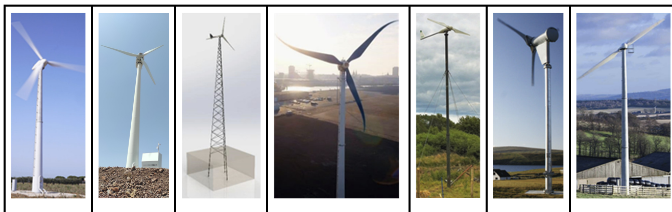
549 Figure 12 - Common HAWT archetypes found in the current DWT market. From left to right: Upwind, active pitch and yaw (photo 550 credit: Tozzi Nord); upwind, stall-controlled and active yaw (photo credit: Eunice); upwind, stall-controlled and tailed passive yaw 551 (photo credit: NREL pix 49511); downwind, stall-controlled, passive yaw (photo credit: Eocycle – formerly XANT); upwind, tailed 552 passive yaw, furling (photo credit: Bornay); downwind, pitch or pitch-coning controlled, passive yaw (photo credit: SD Wind 553 [formerly Proven]); downwind, stall-controlled, passive yaw and teeter (photo credit: Ryse Energy [formerly Gaia]).
