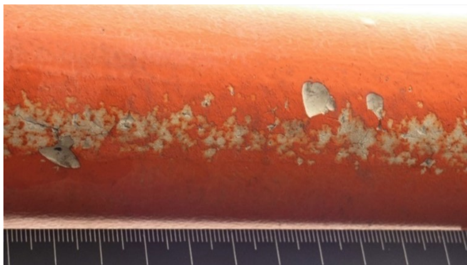
Figure 17. LEE damage on the tip section of a WTB, photographed by TNO
