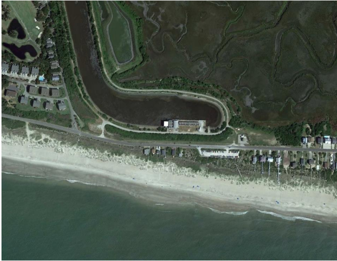
470 Figure 8. Possible location for export cable landfall adjacent to the coolant canal for Brunswick Nuclear Power Plant. Environmental constraints would be minimal here due to the already developed/engineered nature of the location. Source: NOAA.
