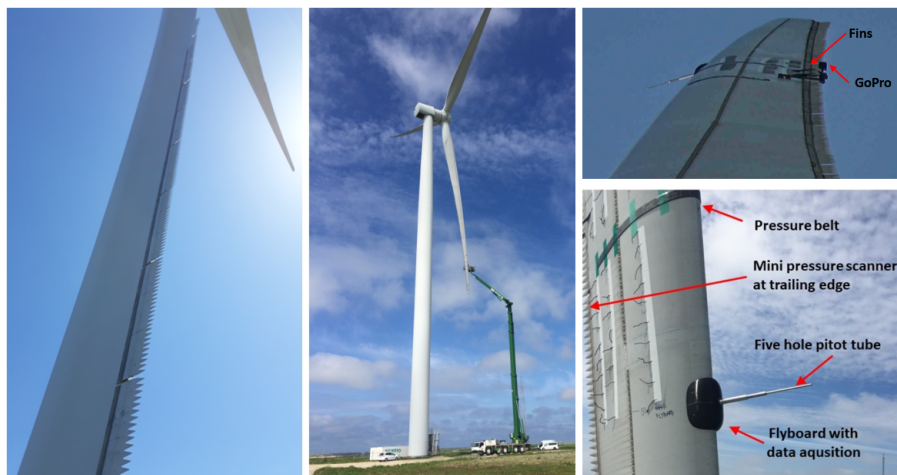
Figure 1. Left photo: Active flap placed on the trailing edge of the blade of the SWT-DD-120 turbine at the Høvsøre test field. Central photo: installation of the flyboard and pressure belt in June 2020. Bottom right photo: close look at the flyboard and the pressure belt. Top right photo: Camera and fins installed to measure the flap deflection. Photos courtesy of SGRE and DTU
