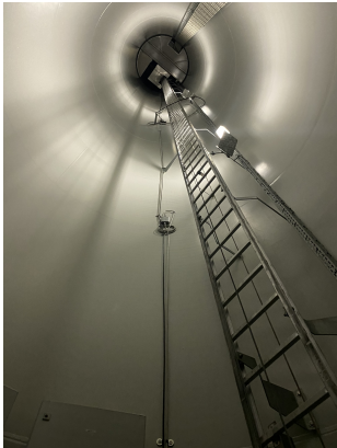
Figure 5. S-Morpho Installation in the Tower.
