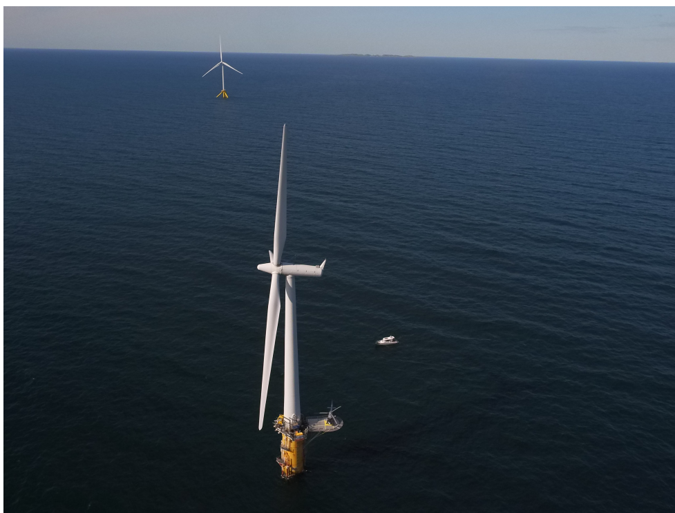
Figure 4. The Zephyros floating offshore wind turbine relies on a Siemens 2.3-MW. Credits: Unitech Energy Group
