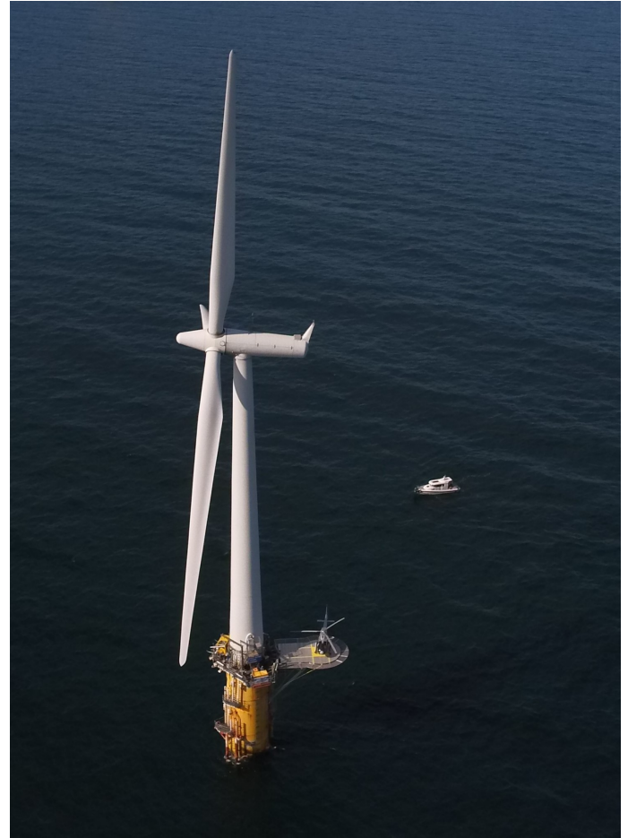
Figure 1. Zephyros, the world's first multi-megawatt FOWT UNITECH (2022). Credits: Unitech Energy Group
