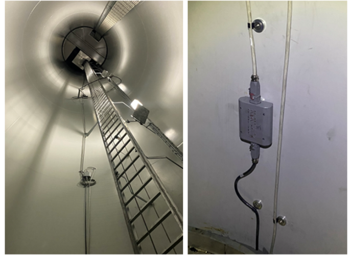
Figure 2. Sensor position along the tower.
