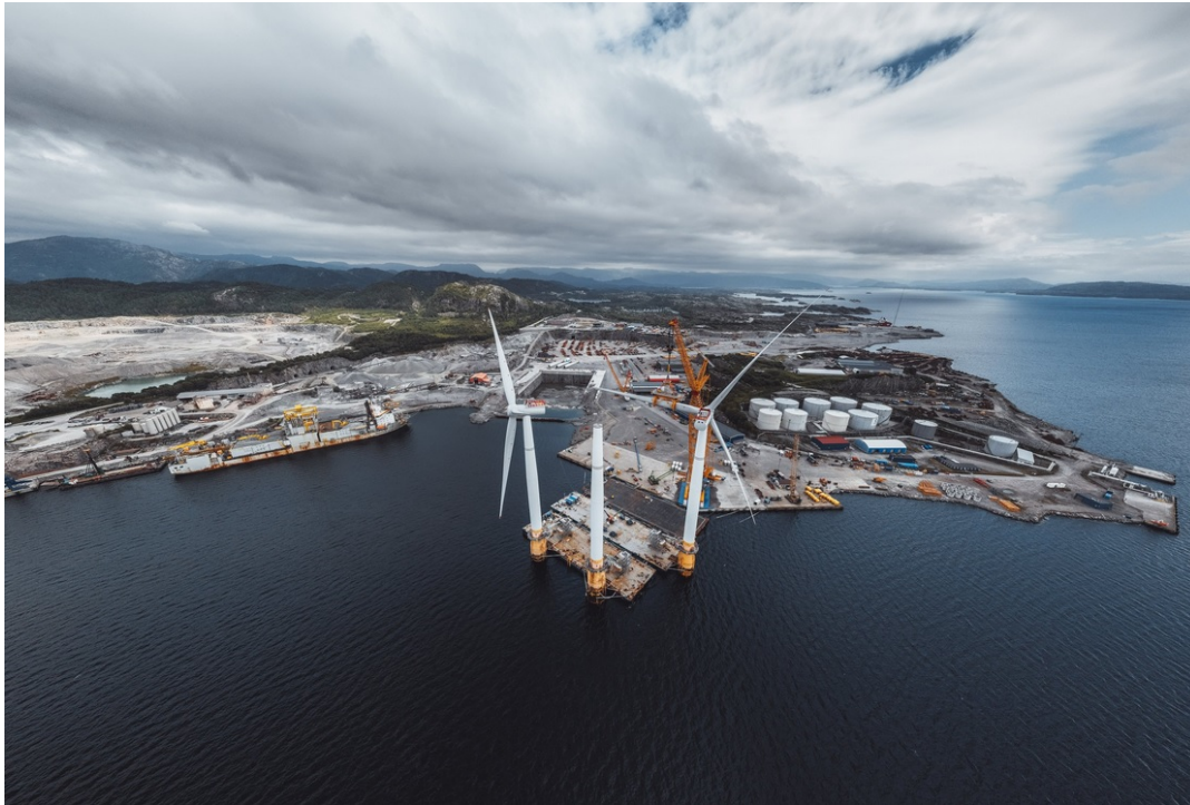
Figure 4. Maintenance of floating offshore wind turbines at shore, in Norway (Source: Wergeland (Wer)).
