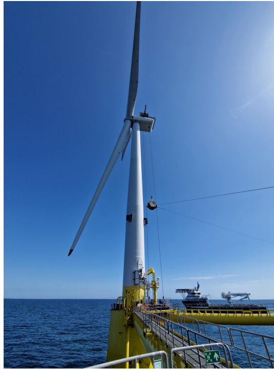
Figure 5. Major component exchange with the help of a a GenHook™ up-tower crane, at the Kincardine offshore wind turbine, on site, south of Aberdeen (Source: Offshore Channel (OffshoreWind.biz by A. Memija, 2024)).
