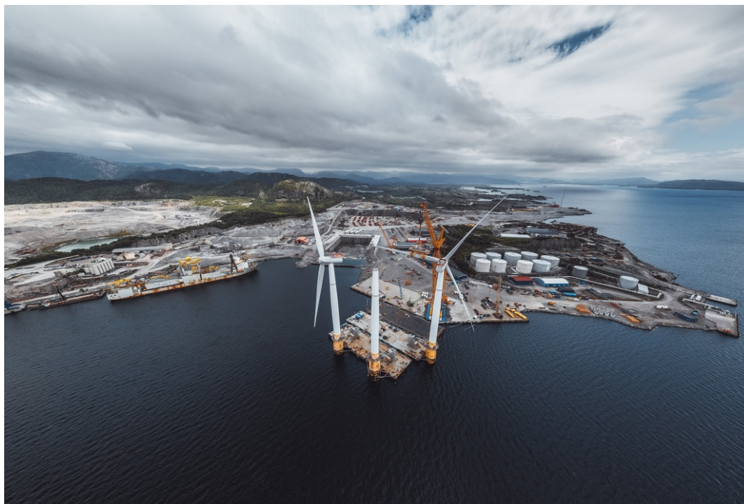
Figure 3. Maintenance of floating offshore wind turbines at shore, in Norway (Source: Wergeland (Wer)).
