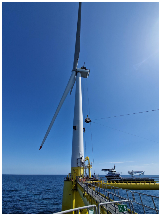
Figure 4. Major component exchange with the help of a GenHook™ up-tower crane, at the Kincardine offshore wind turbine, on site, south of Aberdeen (Source: Offshore Channel (OffshoreWind.biz by A. Memija, 2024)).
