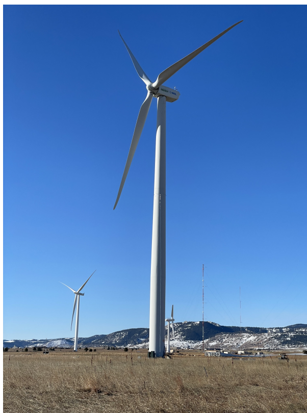
Figure 1. GE 1.5 MW wind turbine located on site 4.0 at the Flatirons Campus, with the rotor in an idling downwind configuration. Photo credit: Rafael Mudafort, NREL.
