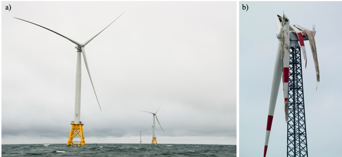
Figure 1: a) Offshore 6-MW wind turbines with 73.5 m-long blades (photo by Dennis Schroeder, NLR/DOE), b) blade failure in a generic wind turbine (photo by Dietmar Händel, CC BY 2.0 license).
