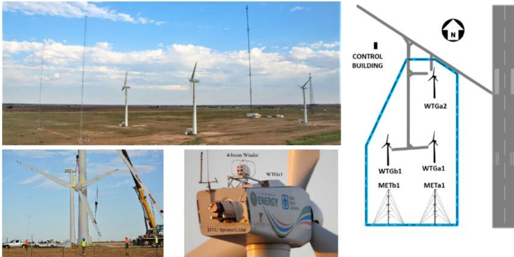
Figure 6 - SWIFT Facilities SNL Texas USA
