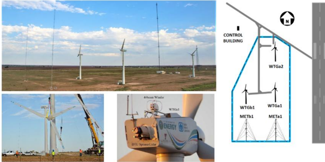
Figure 6 - SWIFT Facilities SNL Texas USA
